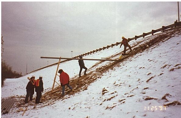
Above: Bore-Gard PVC pipe is being installed on a 45 degree slope near the intersection of Ohio Interstate 271 and Route 480 near Cleveland. Two 220 ft. installations were made about 20 feet apart under the active highway. In spite of the challenging terrain, the pipes were easily assembled and locked together before being installed.
