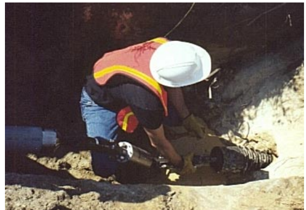
Above Left: In the foreground is the drill entrance location of the straight bore under the street for a total of 100 feet. Above Right: A close-up look at the pulling eye (left), swivels, on-board computer and 6 inch reamer (right) attached to the lead end of the Bore-Gard pipe (left) as it enters the ground.
