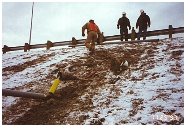
Above Left: The 8 inch diameter reamer is seen here along with the strain gauge and on-board computer used to measure the pull force on the pipe. An expandable pulling eye was used to grip the leading end of the pipe. Above Right: The directional boring machine and a 1,200 gallon water tank.
