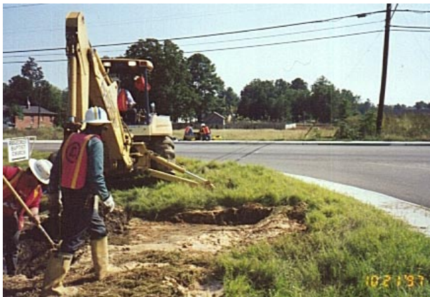
Above Left: In the foreground is the drill entrance location of the straight bore under the street for a total of 100 feet. Above Right: A close-up look at the pulling eye (left), swivels, on-board computer and 6 inch reamer (right) attached to the lead end of the Bore-Gard pipe (left) as it enters the ground.
