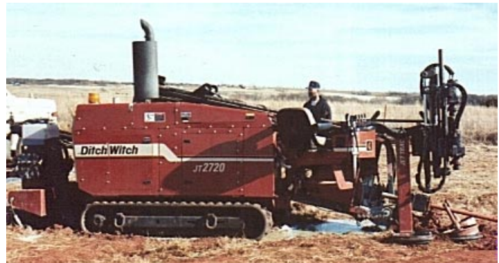
At Left: In the foreground is the reamer attached to the drill string. Barely visible from 1,000 feet on the horizon is the drilling machine. Above Right: A close-up look at the powerful Ditch Witch ® JT2720 that quickly and easily pulled in the 1,000 ft. string of Bore-Gard.
