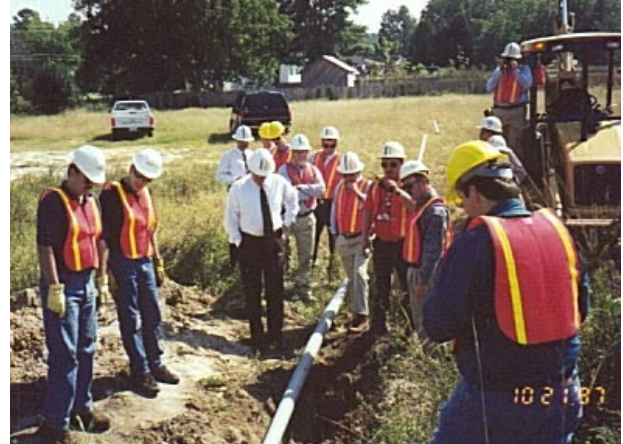
Above Left: Bore-Gard PVC pipe at a depth of 6 feet is being pulled beneath the active roadway. The tight transition and resultant bend radius was no problem for the strong joint design. Above Right: The entire Telco company crew was impressed with the simplicity, fast assembly, and strength of Bore-Gard. The entire 100 feet of pipe was laid out in a few minutes for before the installation.
