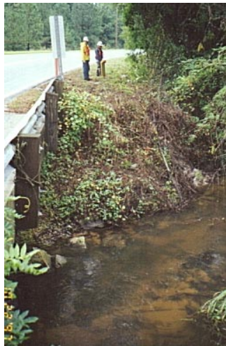
Far Left: At the entrance pit, Bore-Gard PVC pipe is being pulled into the 6 inch reamed hole through challenging tree roots, rock, clay and sandy soil. Left: Facing the entrance pit overlooking a creek 6 ft. below road level. Maximum depth of 16 ft. was reached below the creek bed. Space restrictions required the pipe to be added every 20 feet of the bore. The simple joint design enabled quick assembly to easily keep pace with pulling of the reamer.
