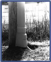
Steel U-Guard required grounding, strapping, and does not have belled ends.
